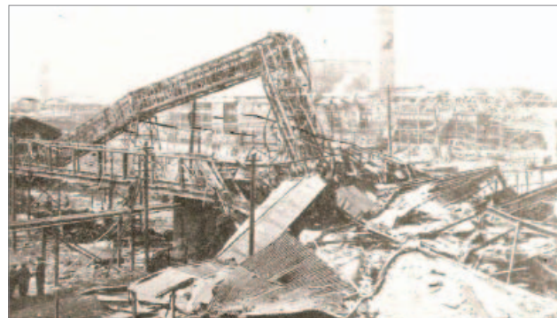
Aftermath of the Chilwell Explosion
