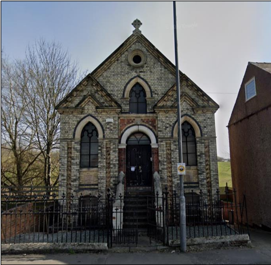
Front Elevation of the Chapel (Photo Credit: Google Maps)
