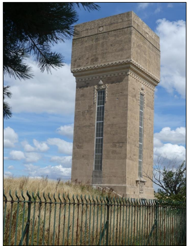
Swingate Water Tower in 2022. Photo Credit: Steve Arundel
